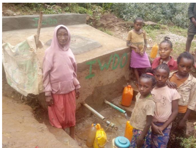
These are simple wells. The spring water at the foot of afforested mountains is collected and piped to the wells. This allows people to fill their canisters with fresh, clean drinking water.
