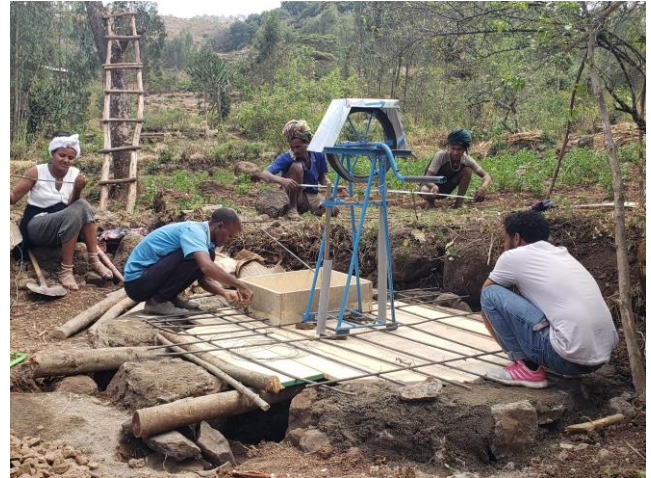
Thanks to rising groundwater levels at the foot of afforestation areas, water can be pumped up manually from shallow depths using 'Rope Water Pumps' and does not have to be carried over long distances on foot in canisters.
