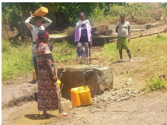
These are simple wells. The spring water at the foot of afforested mountains is collected and piped to the wells. This allows people to fill their canisters with fresh, clean drinking water.
