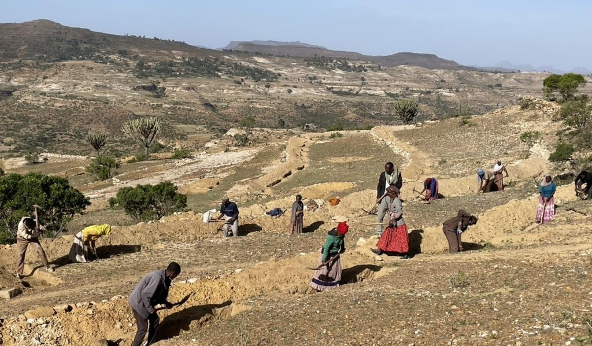
Soil and water conservation: construction of terraces in the lower part.
