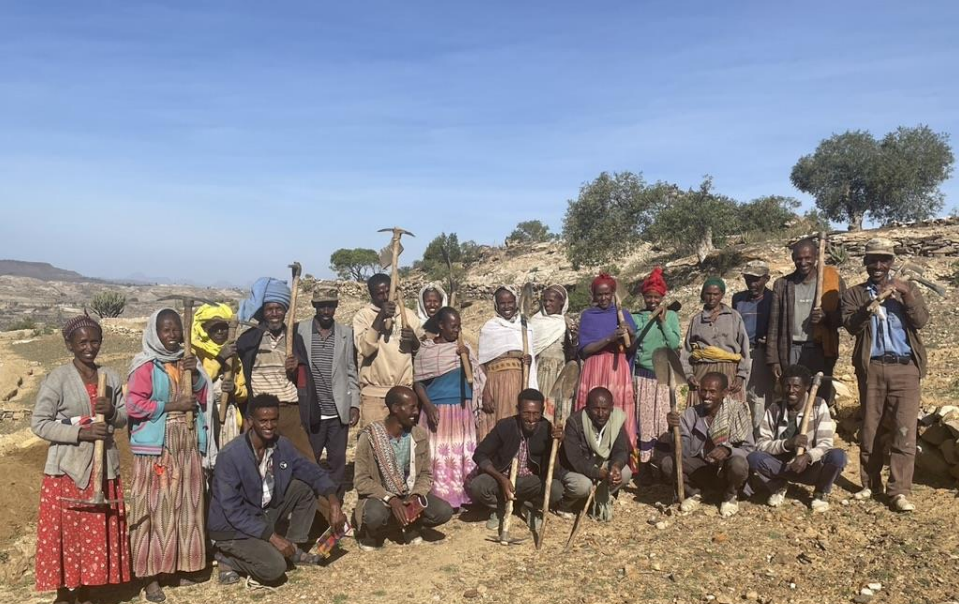
Beneficiary farmers constructing terraces.
