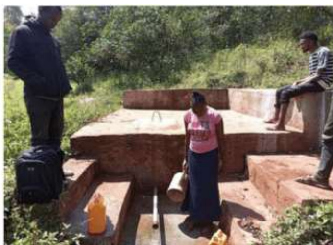
At the foot of reforested mountains, water is stored in well chambers (which was a very common practice in Switzerland before bigger tanks have been built). Fresh and cleanly filtered drinking water is therefore also available during droughts.
