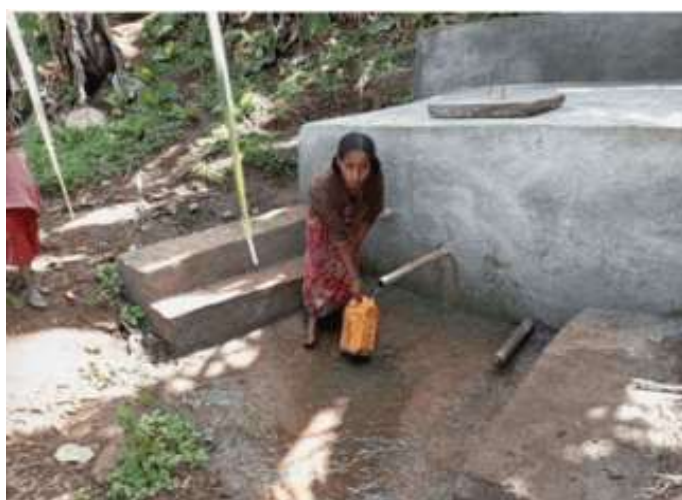
At the foot of reforested mountains, water is stored in well chambers (which was a very common practice in Switzerland before bigger tanks have been built). Fresh and cleanly filtered drinking water is therefore also available during droughts.
